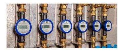
PoC: digital water meter with acoustic noise detection
